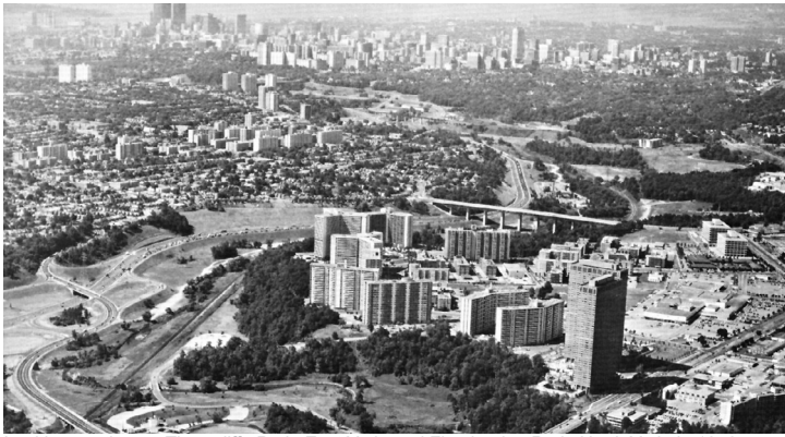
Looking south over Thorncliffe Park, East York, and Flemingdon Park, North York, in 1970 - courtesy Archives of Lockwood Survey Corporation Limited.
