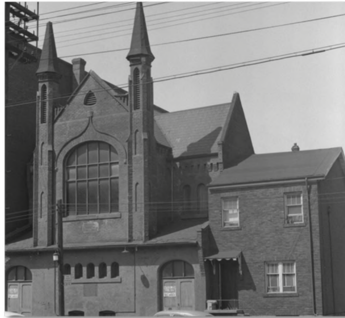
1953 PHOTOGRAPHER: J.V. SALMON, AGO FOYER. Photograph of the church's street facade from 1953.
