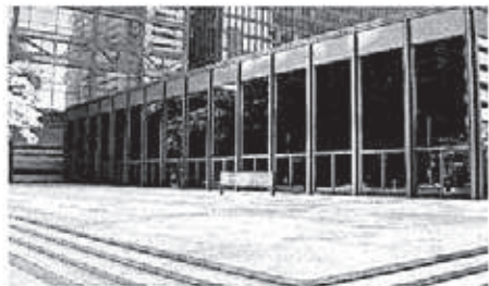
The Toronto Dominion Centre on Bay Street designed by Mies van der Rohe and Parkin exemplifies the International Style refinement and sparsity.
