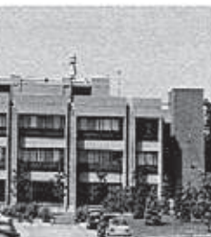
the York University Campus was on, Parkin, Shore and Moffat.
