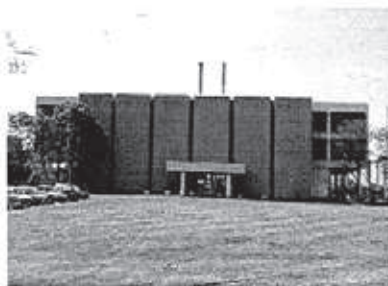
The south facing front elevation with its projecting bays, house the building services.
