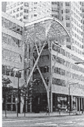
Renowned for its sculptural steel forms, Santiago Calatrava's BCE Place spans the void between various buildings on Bay Street.
