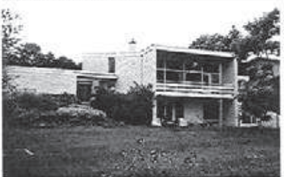
In the rear of the house, framed views of the surrounding site are created along the primary axis.
