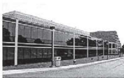
The steel frame office wing was built in 1991 by The Austin Company.
