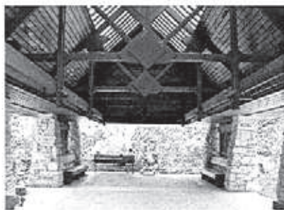
A view of the heavily detailed roof structure.
