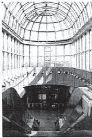
The Yorkdale Subway Station is a Significant North York example of Expressionism.
