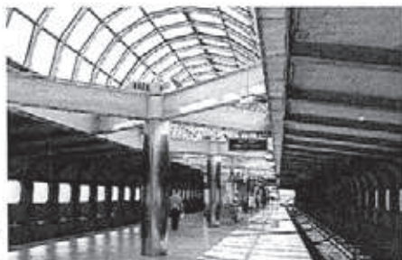
The light filled boarding platform of the Yorkdale Subway Station
