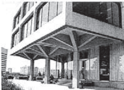
Expressive columns support three sides of the building with their tree-like forms.
