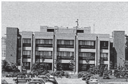
York University Campus offers a wealth of examples of Brutalism seen here in Petrie Sciences Building
