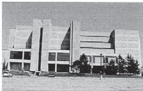
The heavily textured concrete and bold forms of the Scott Library on York University Campus is indicative of the Brutalist Style.
