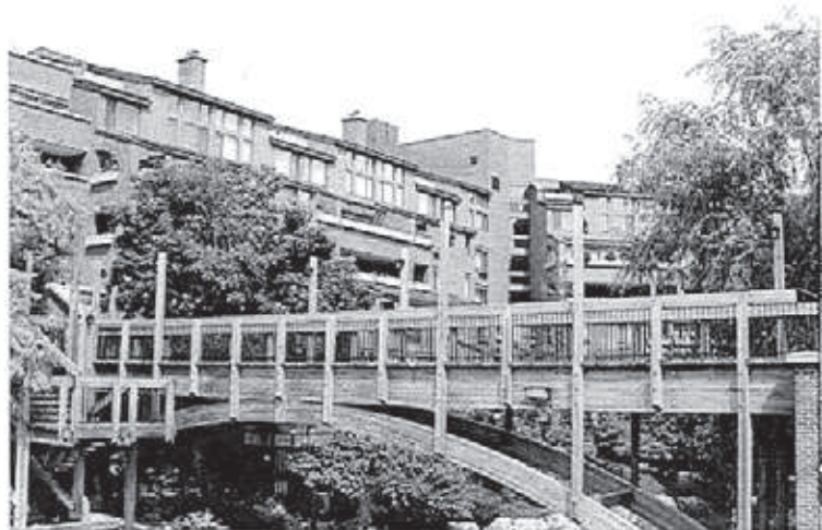
A pedestrian bridge carries pedestrians over a landscaped garden from Avenue Road to the Bedford Glen Housing Development.
