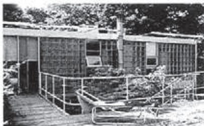
A terrace above the garage is connected by bridges to the bedrooms.
